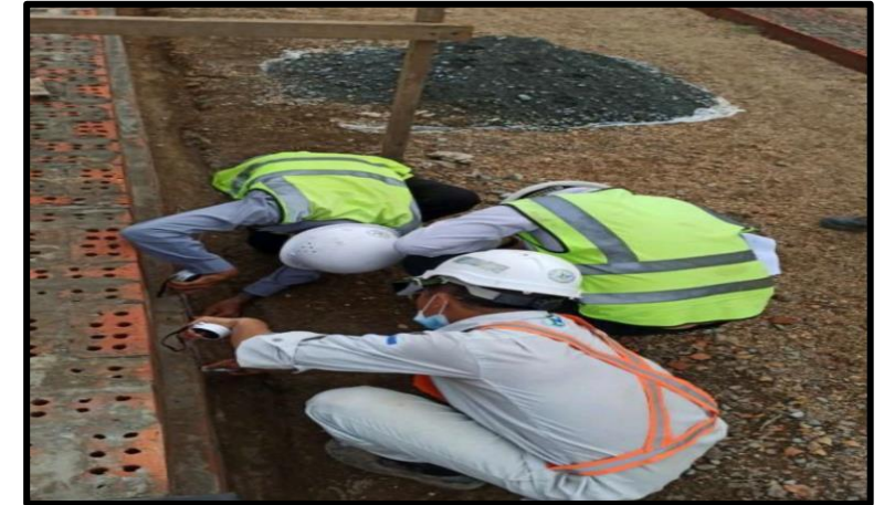
Inspection the completed work activities with consultant parties
